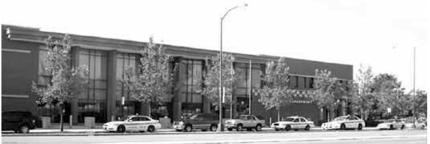
Front of Station
